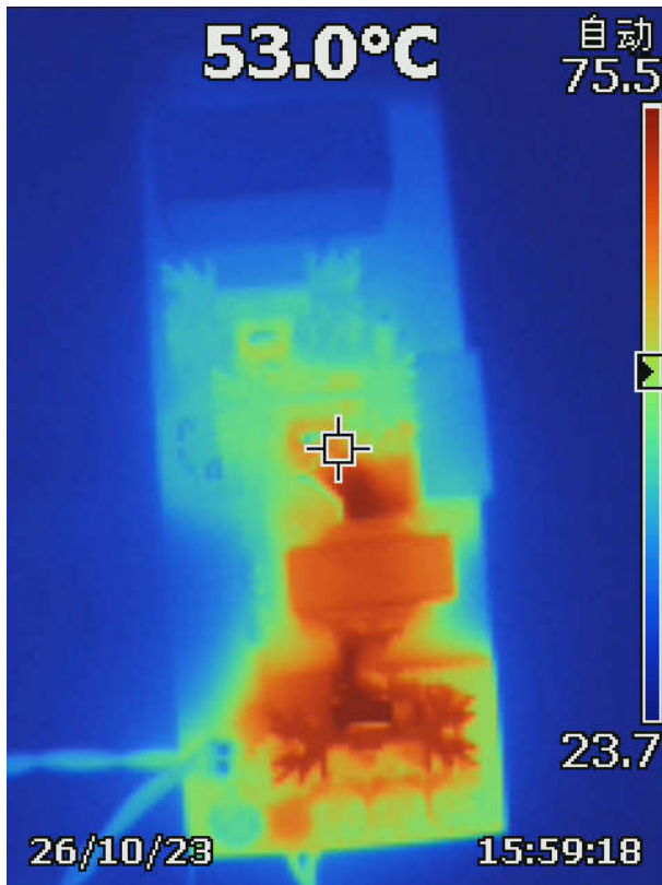
Figure 2-6. Thermal Image 600 V IN 12 V, 4-A Load Top View
