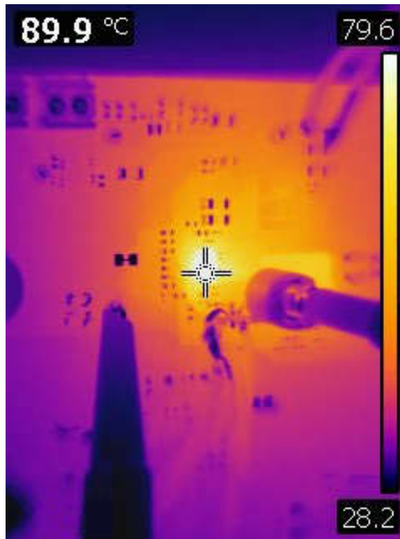
Figure 2-9. Thermal Image at 18 V IN
