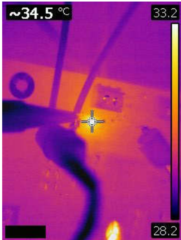
Figure 2-10. Thermal Image at 4.2 V IN , 3.3 V OUT , 0.15A I OUT
