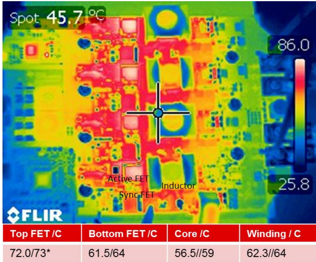
Figure 24 Thermal image of the BidirectionDCDC board on a heat sink performing ZVS Buck operation at 110 A.
