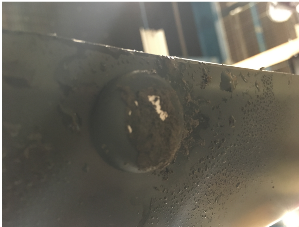
图 59. Mud on Ultrasonic Transducer
